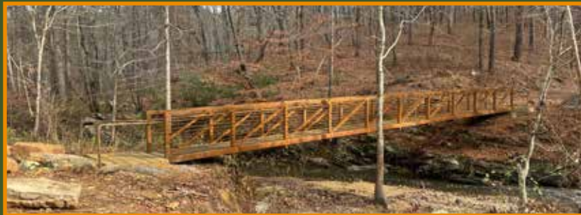
Recently completed bridge at Jogloma-Scott Lake
