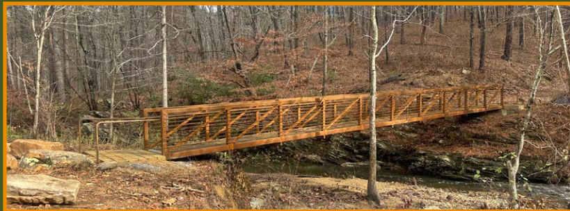
Recently completed bridge at Jogloma-Scott Lake
